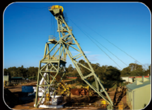
MINE HEAD-FRAME HOISTING INSTALLATION
