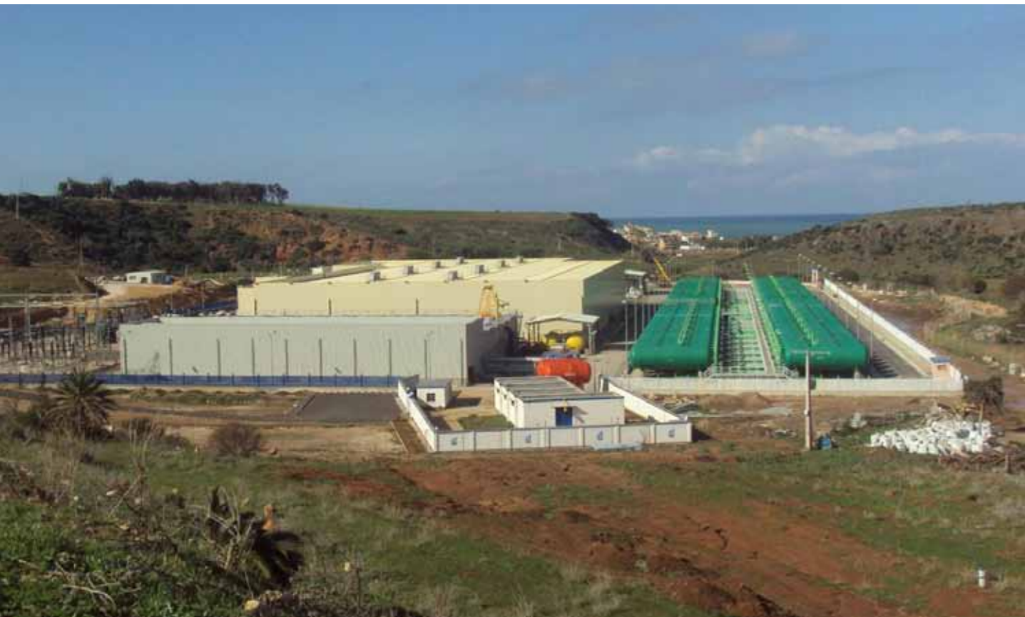
Beni Saf Desalination Plant (Algerie)
