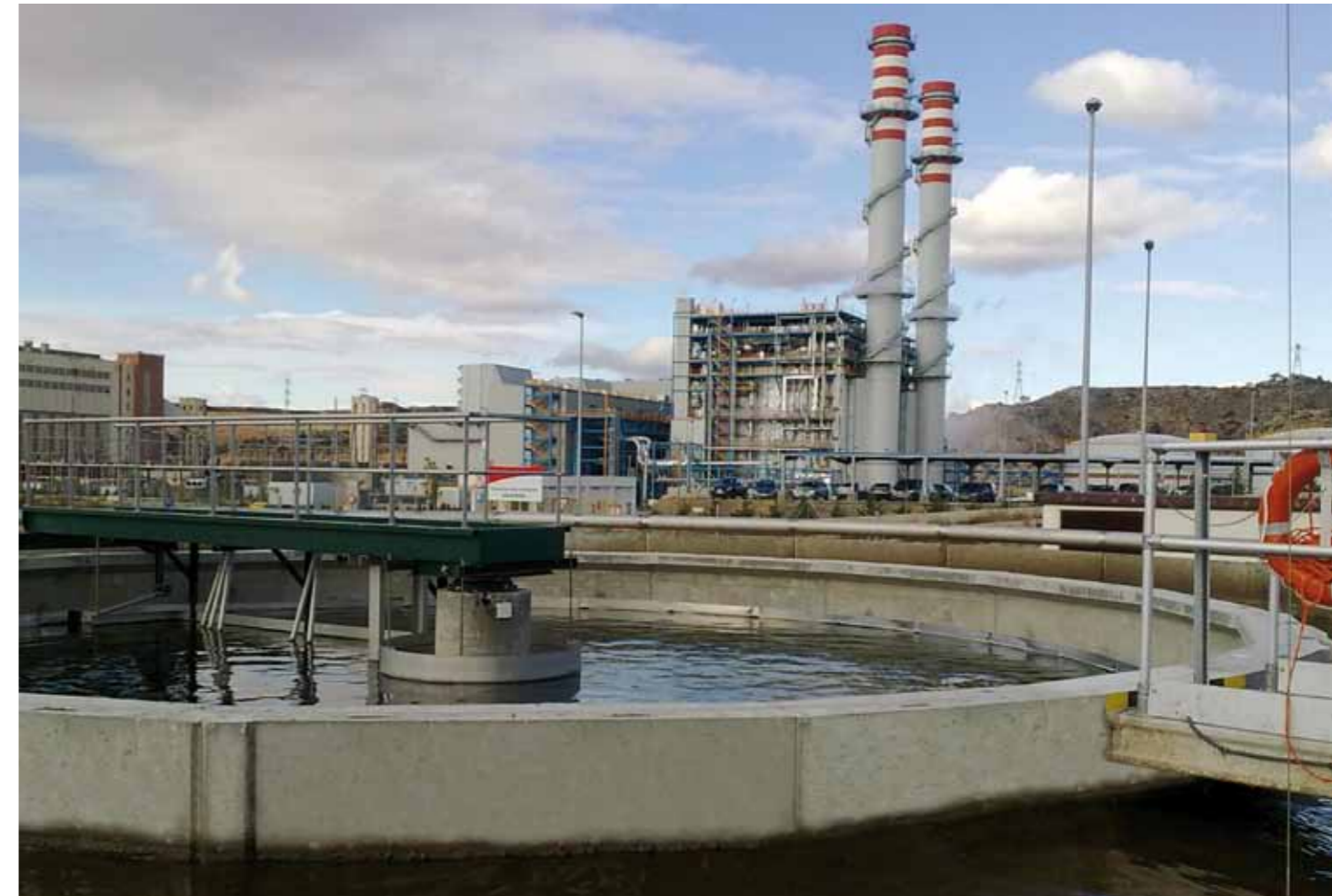
WWTP of the city of Escatrón (Spain) with the Combined Cycle constructed by Cobra Group at the end
