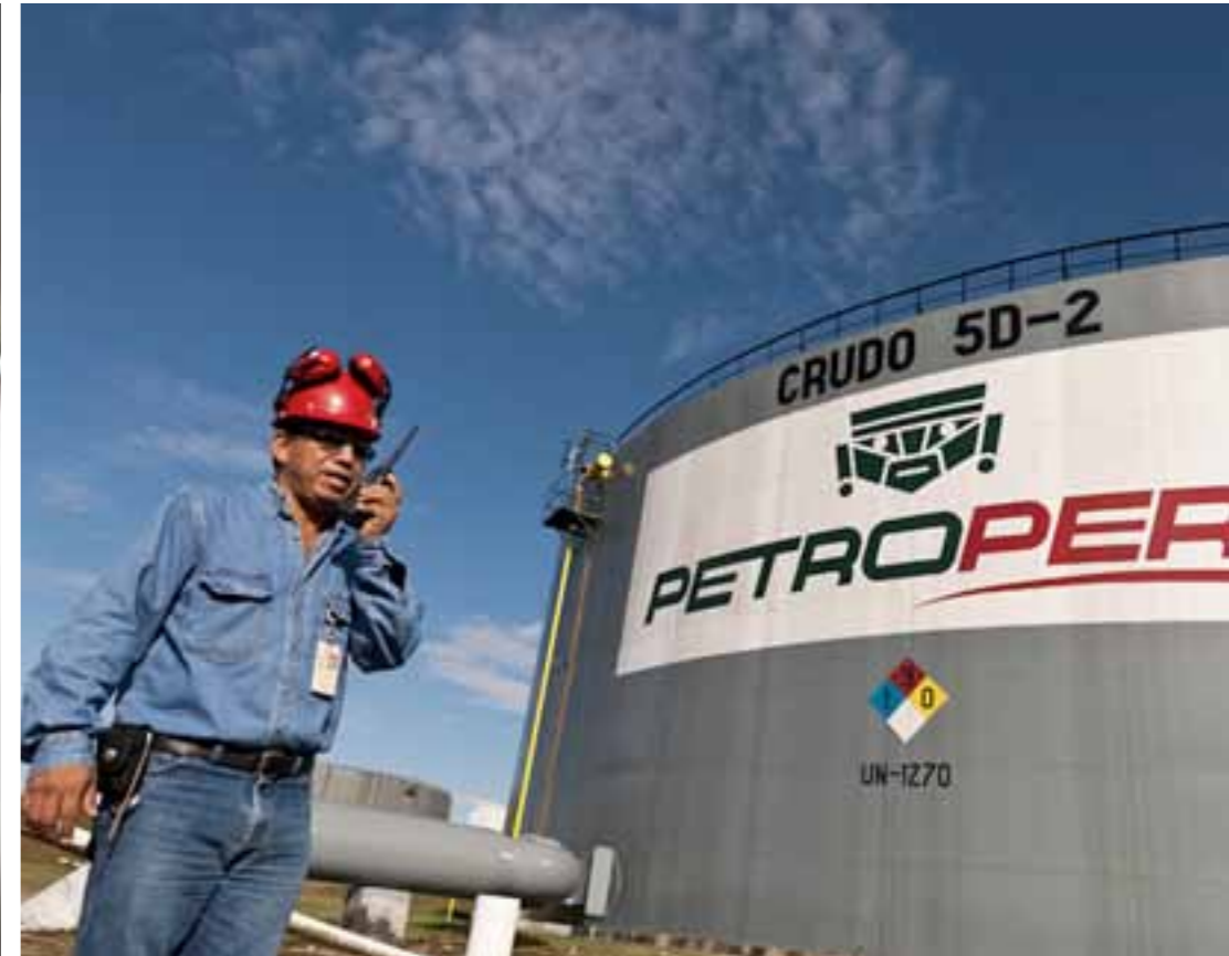
Worker inspecting the pipeline
