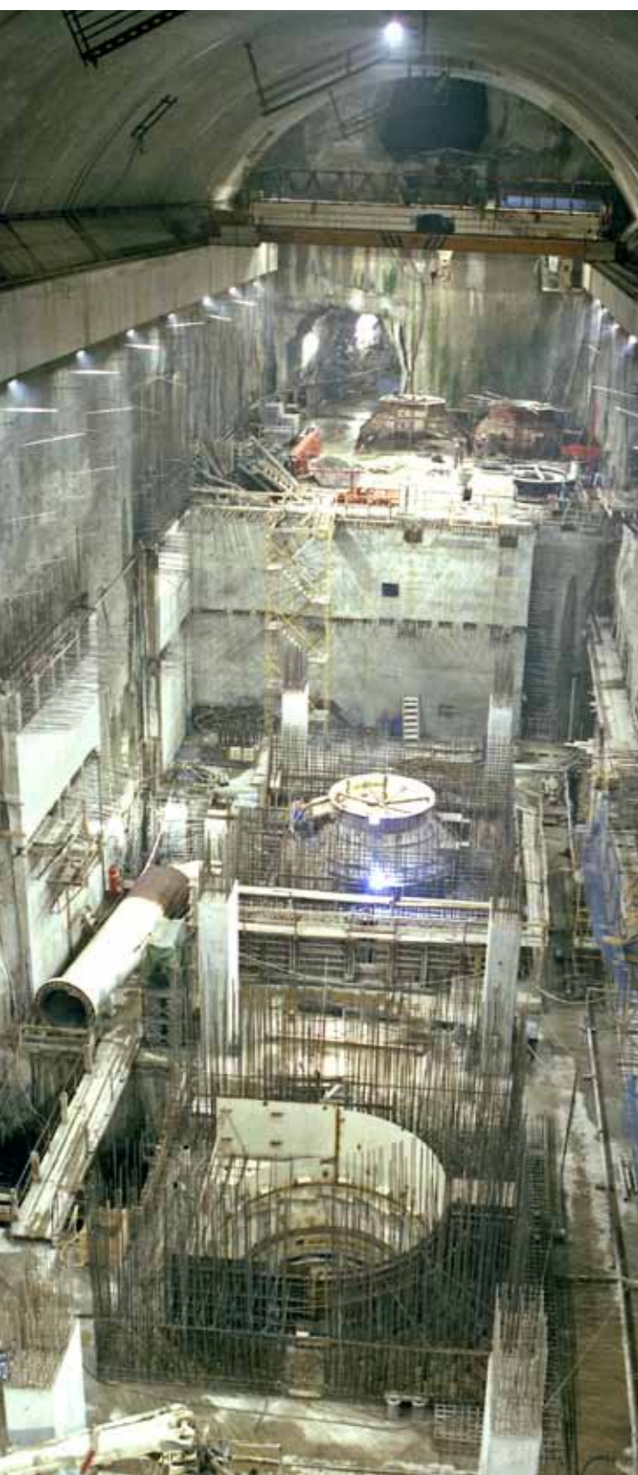
Construction at the Hydro Power Plant, Cortes de Pallás
