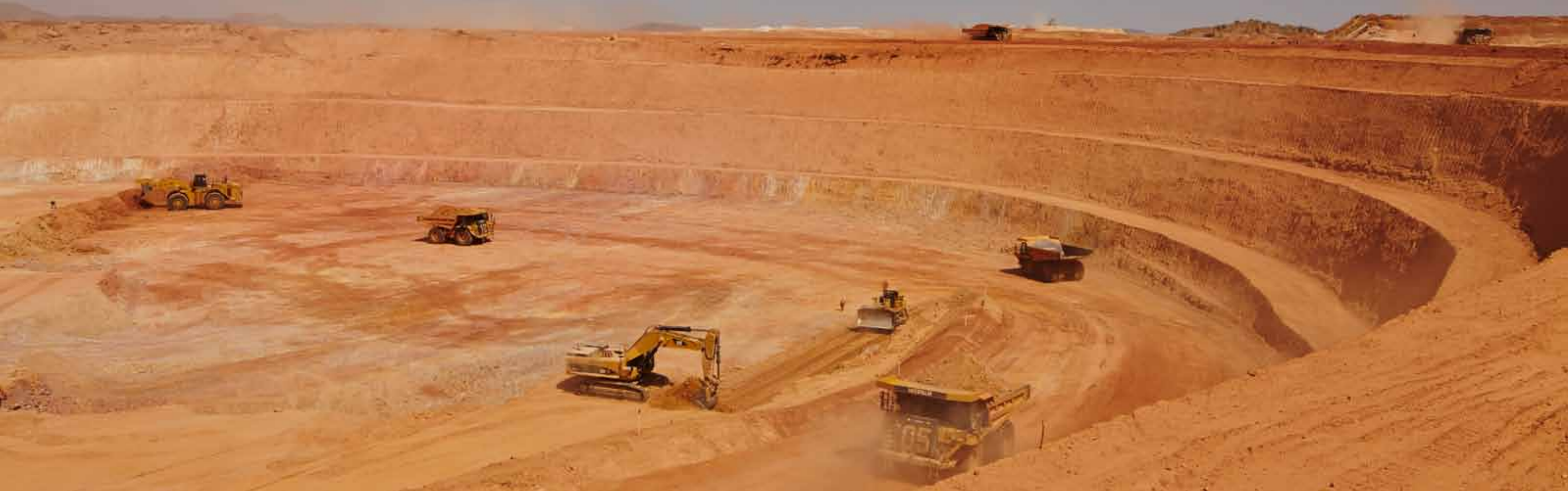
Open pit at Bissa
