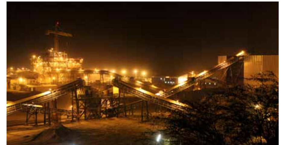
Taparko processing plant
