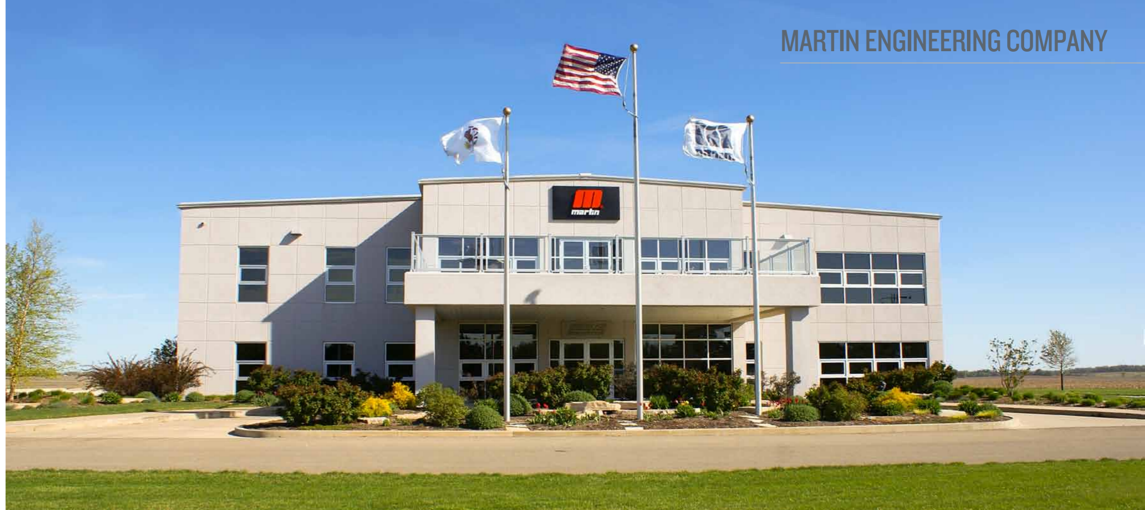
The Center for Innovation (CFI) at Martin's world headquarters in Neponset, Illinois
