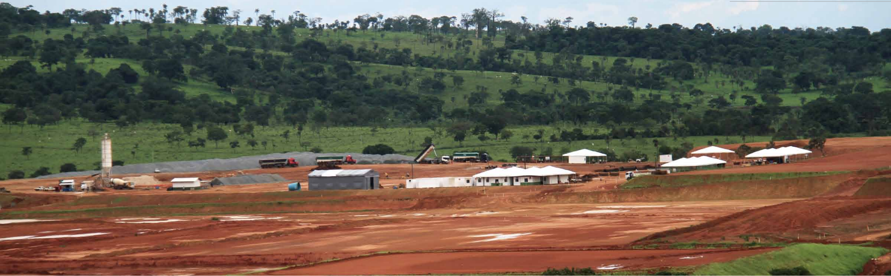
Construction at MBAC's Itafós SSP project
