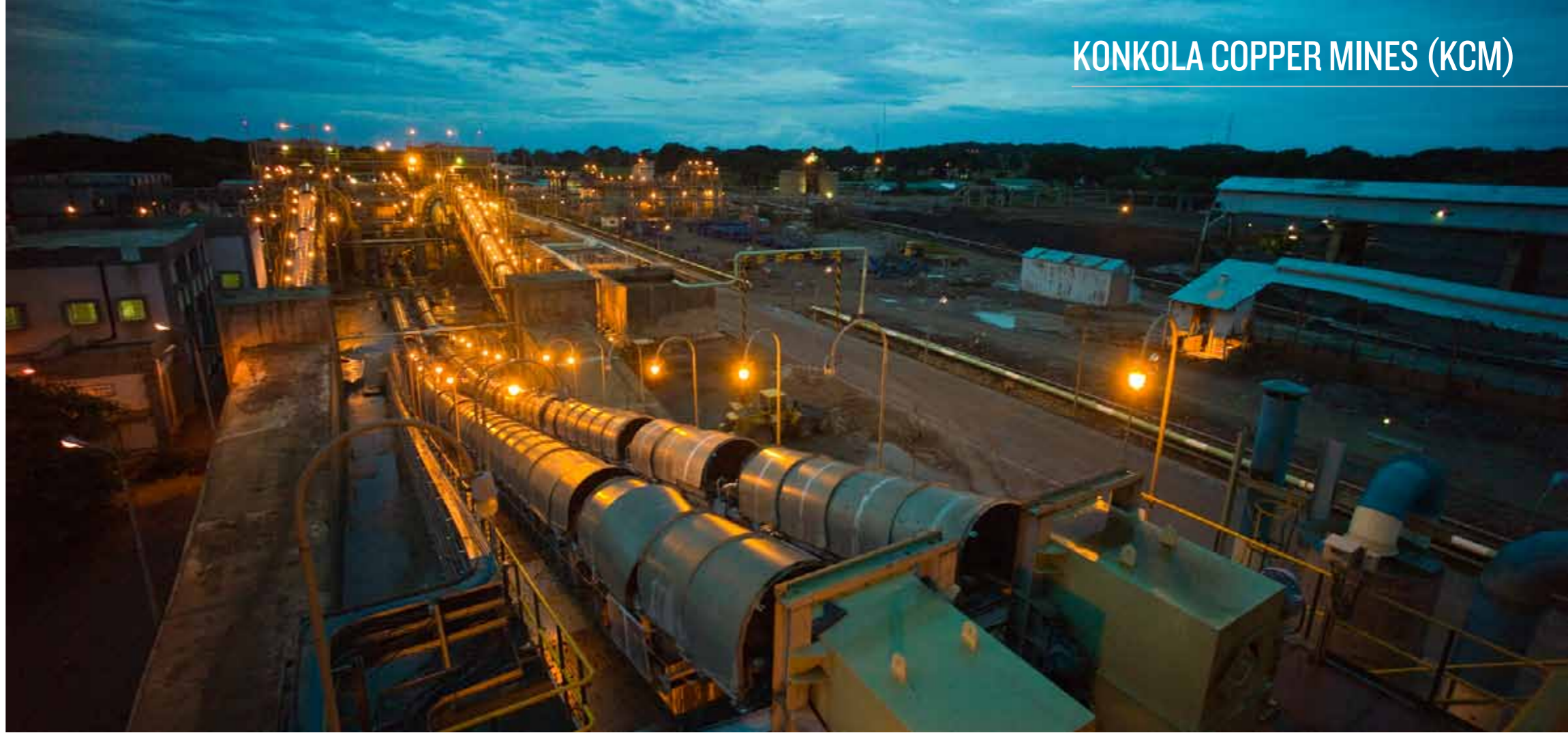
Overview of the plant site
