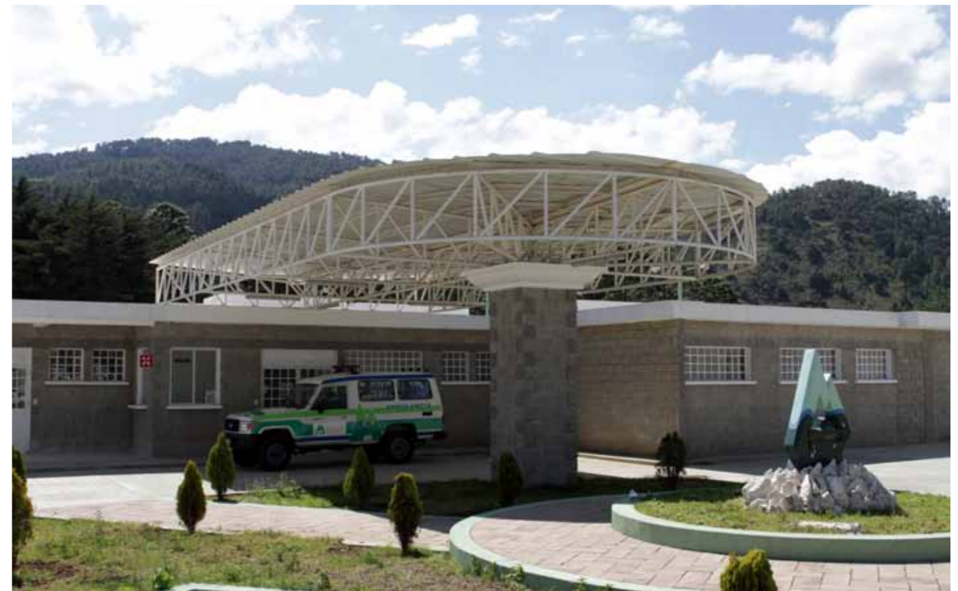
Exterior of the CAP centre
