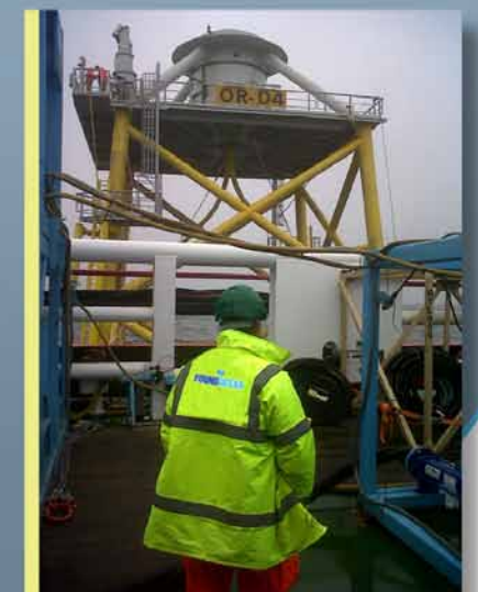
FoundOcean foundation grouting at Ormonde OWF
