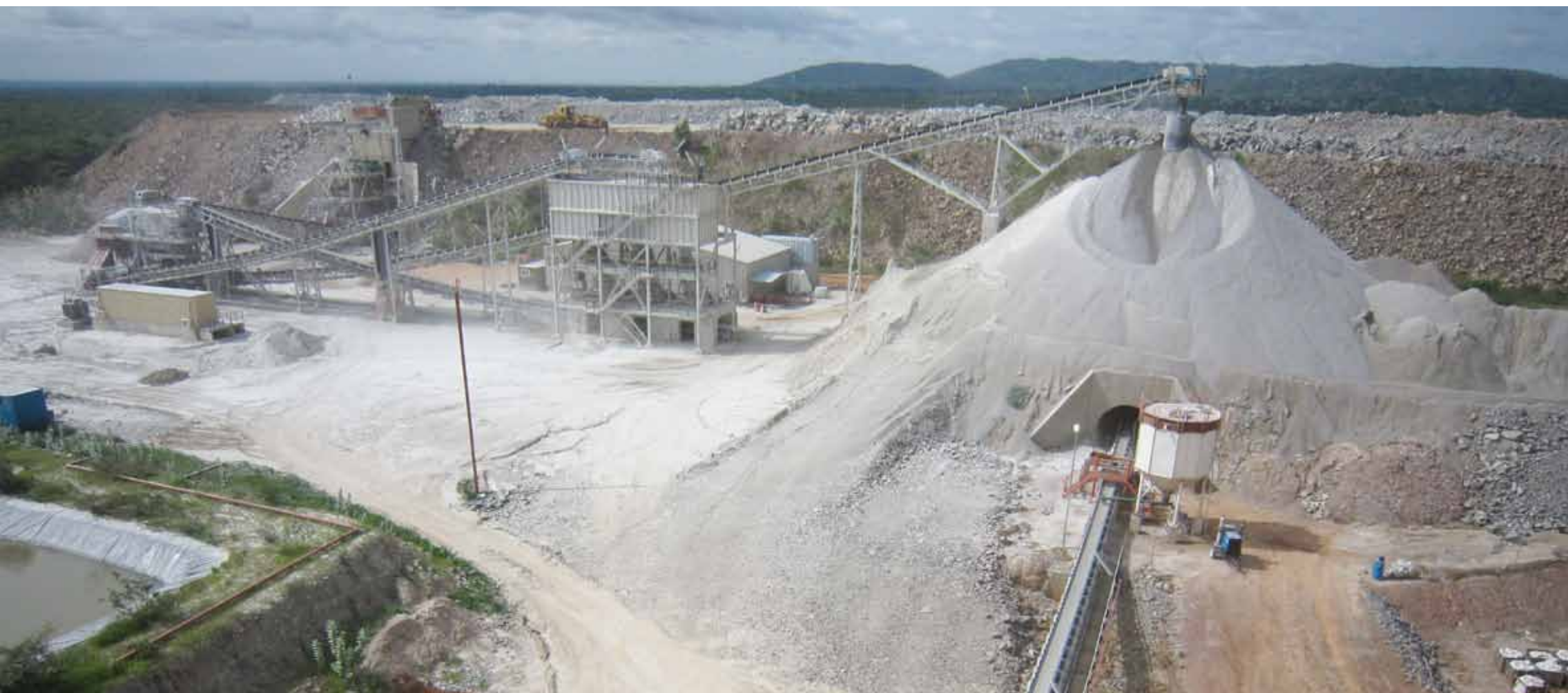
Youga Gold Mine: primary crusher and crushed ore stockpile
