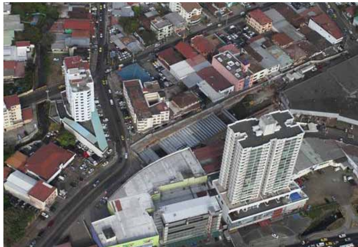
Aerial view of excavation operations
