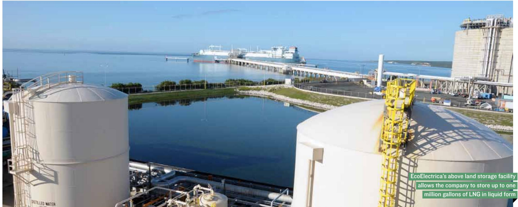
EcoElectrica's above land storage facility allows the company to store up to one million gallons of LNG in liquid form
