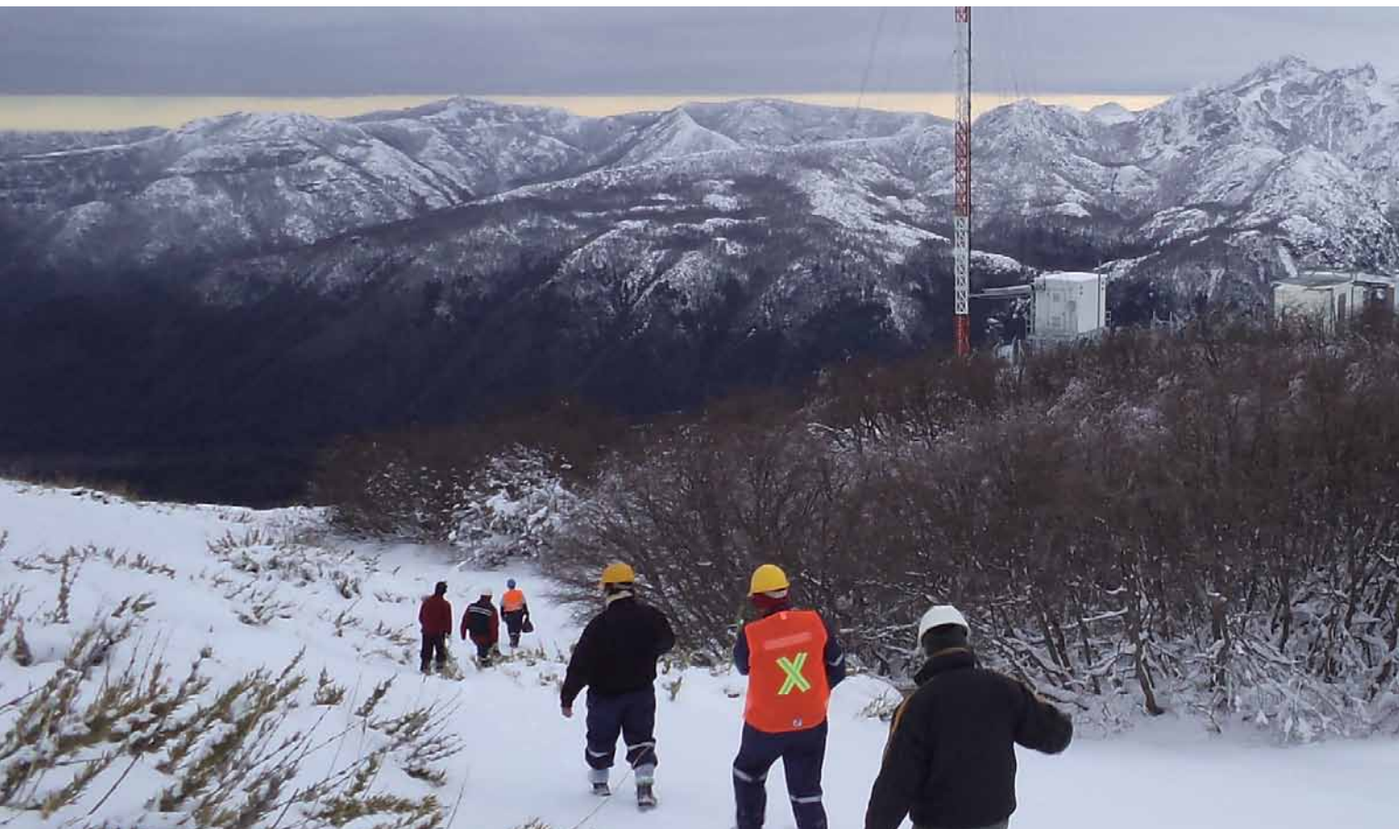
Installation of antenna in the Andes Mountains
