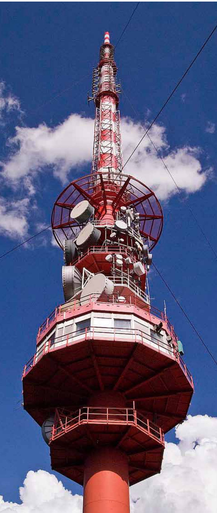
Top of a broadcasting tower
