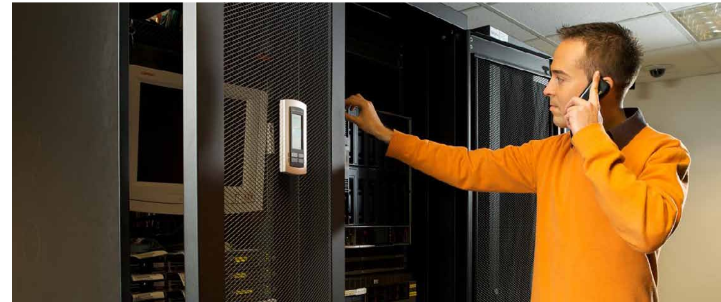
Multiplex - digital broadcasting technology
