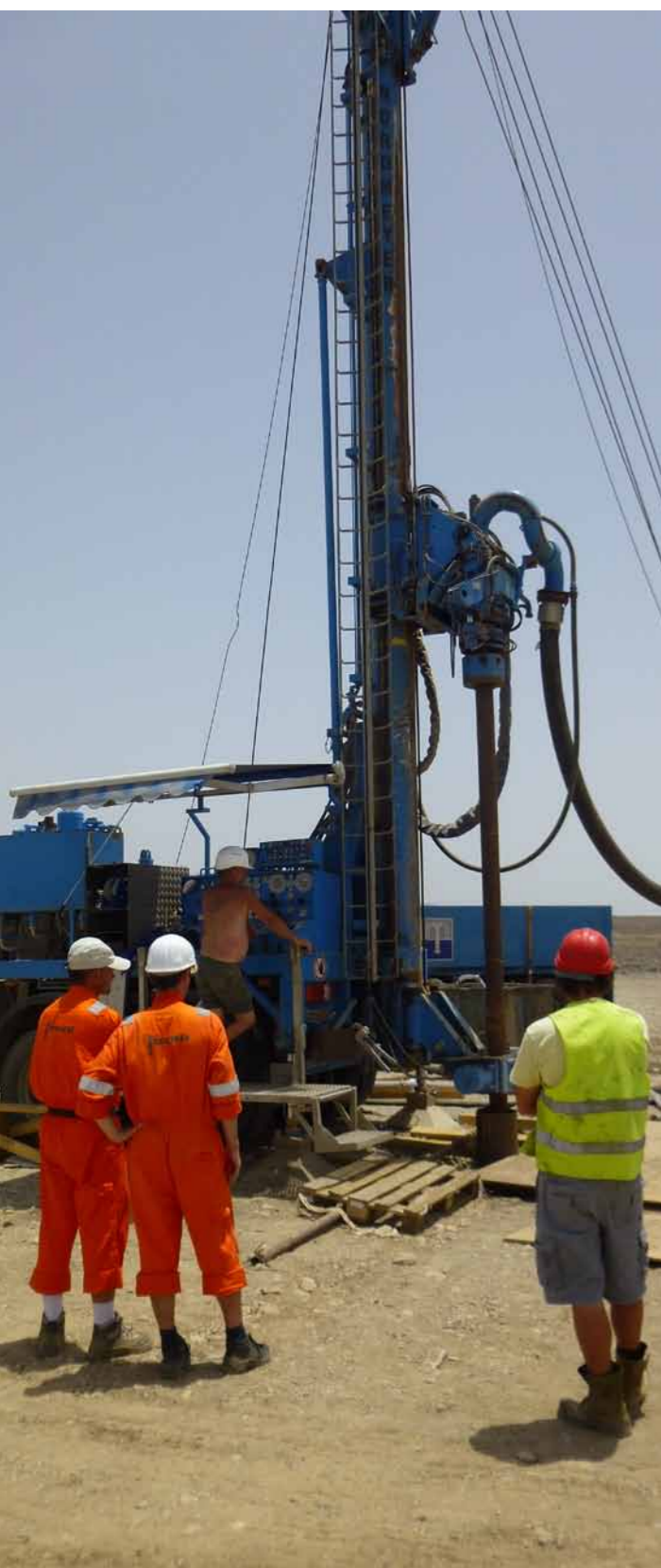
Water well drilling
