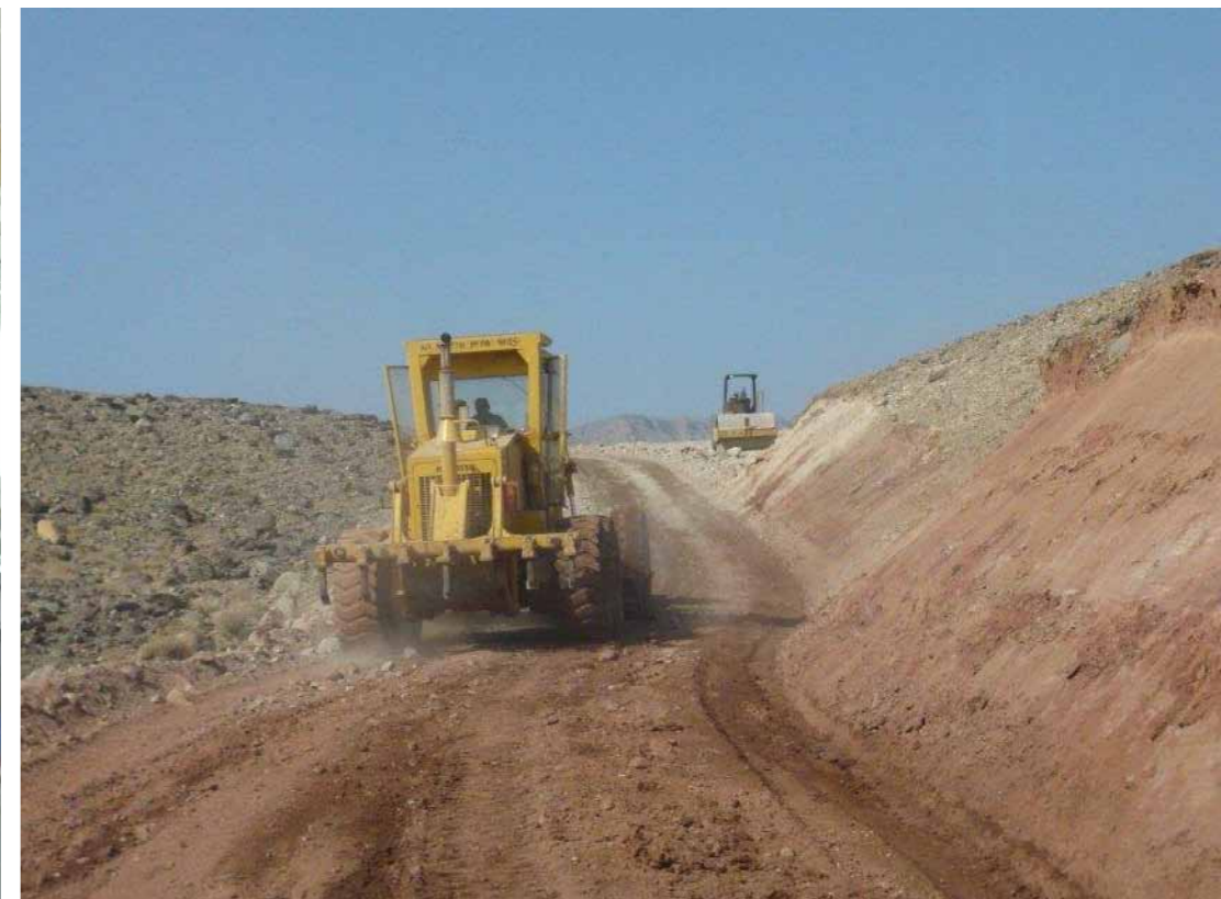
Road rehabilitation work by the government of Ethiopia, Dallol Project
