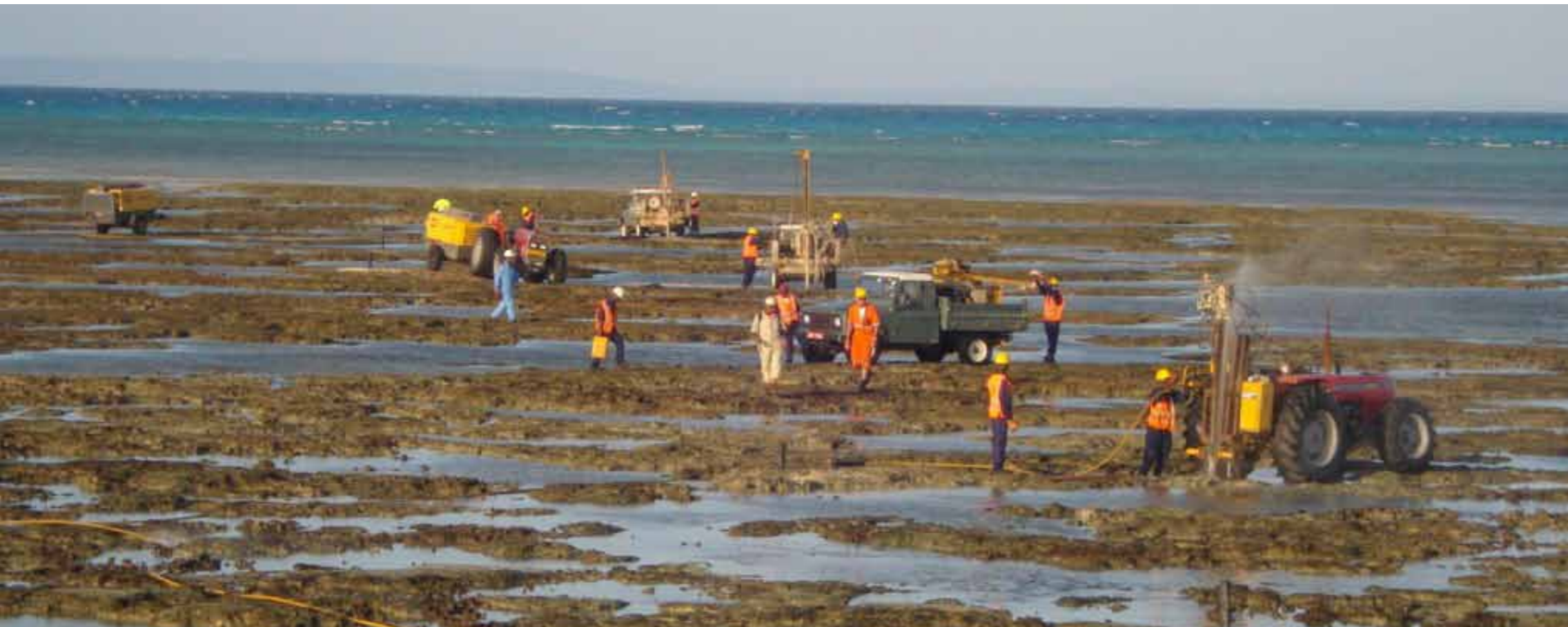
Drilling operations at low tide
