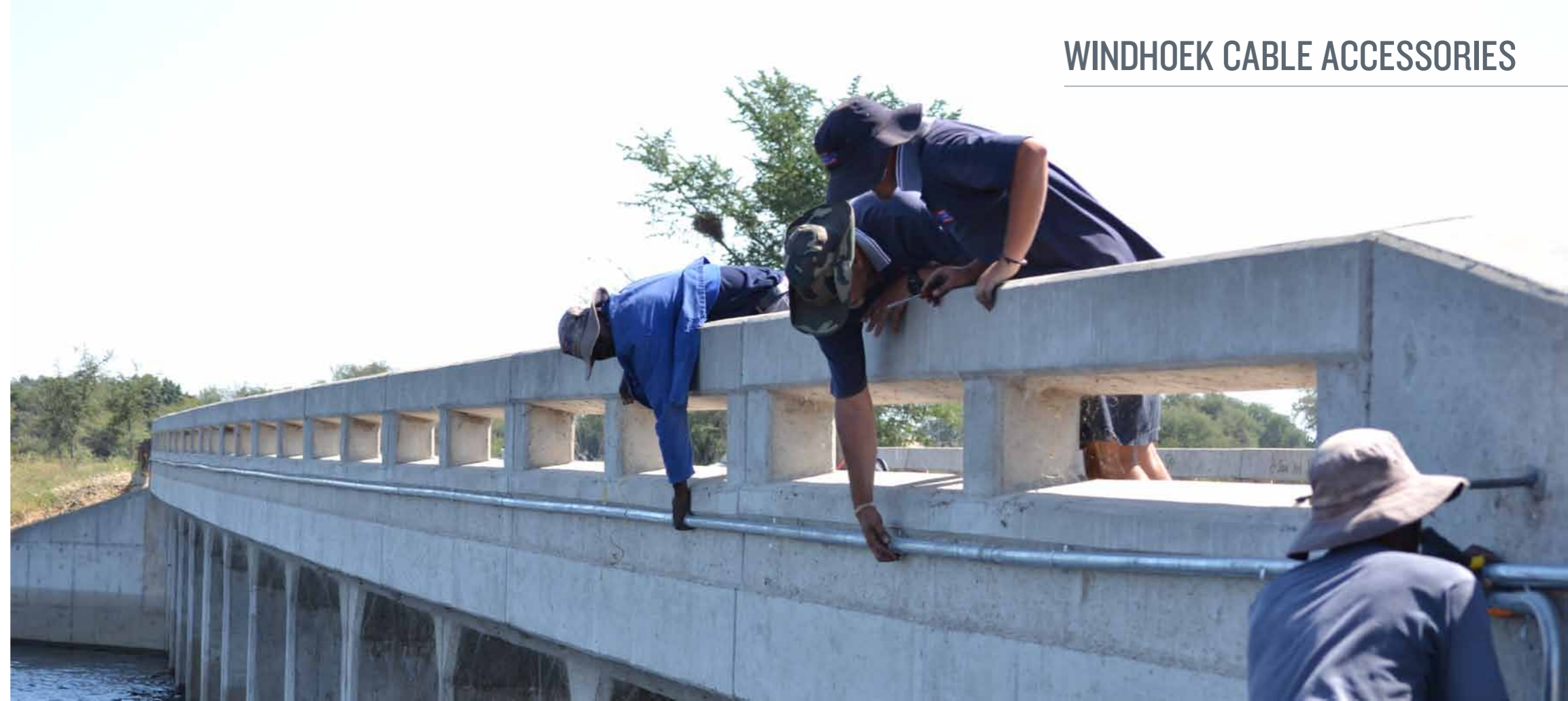
Fibre being installed over Chobe River
