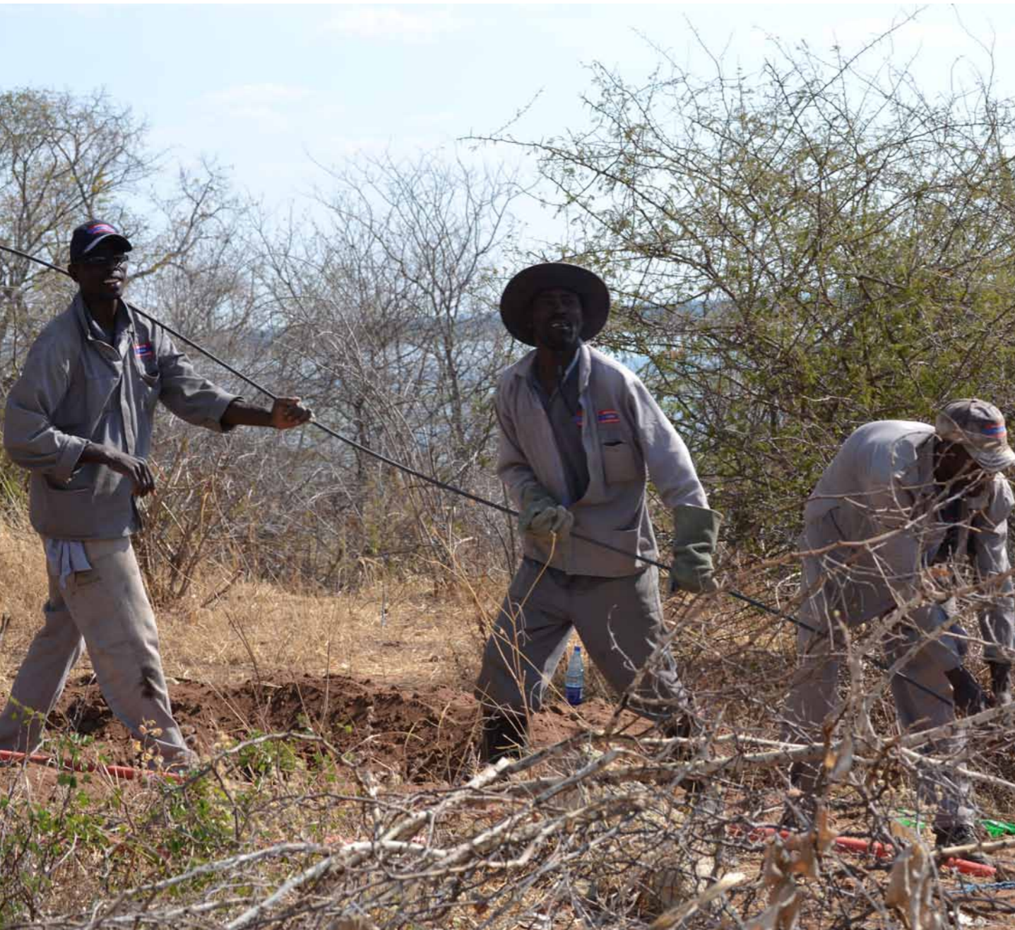
Laying cable in Caprivi Province, Namibia
