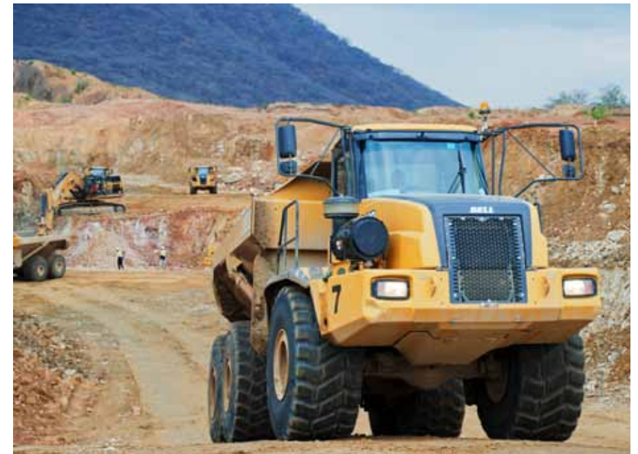
Removing waste from Luika pit
