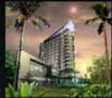
Radisson Hotel Maputo - Mozambique
