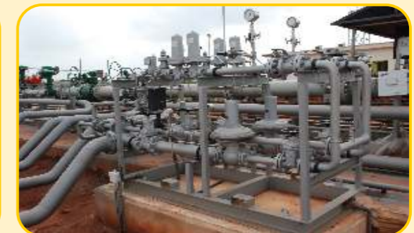
GAS METERING STATION FACILITY OF NIPP LOT 1, BUILT BY OILSERV LIMITED
