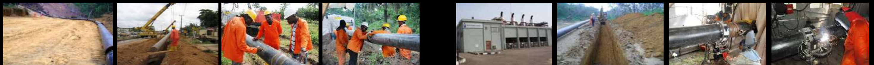
CONSTRUCTION, BUTT WELDING AND VISUAL INSPECTION OF BUTT WELDED GAS PIPELINE JOINT
