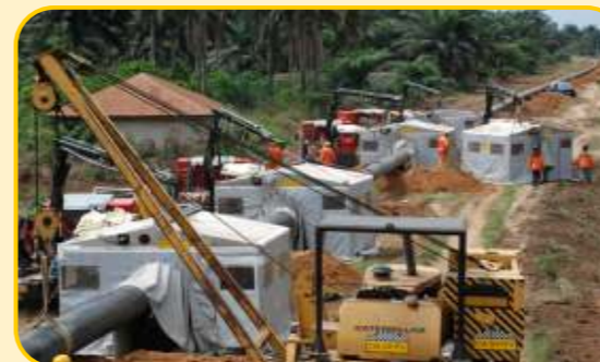
BUTT WELDING OF GAS PIPELINE JOINTS USING OILSERV DIFFERENT AUTOMATIC WELDING STATIONS AND SPECIAL WELDING TENTS
