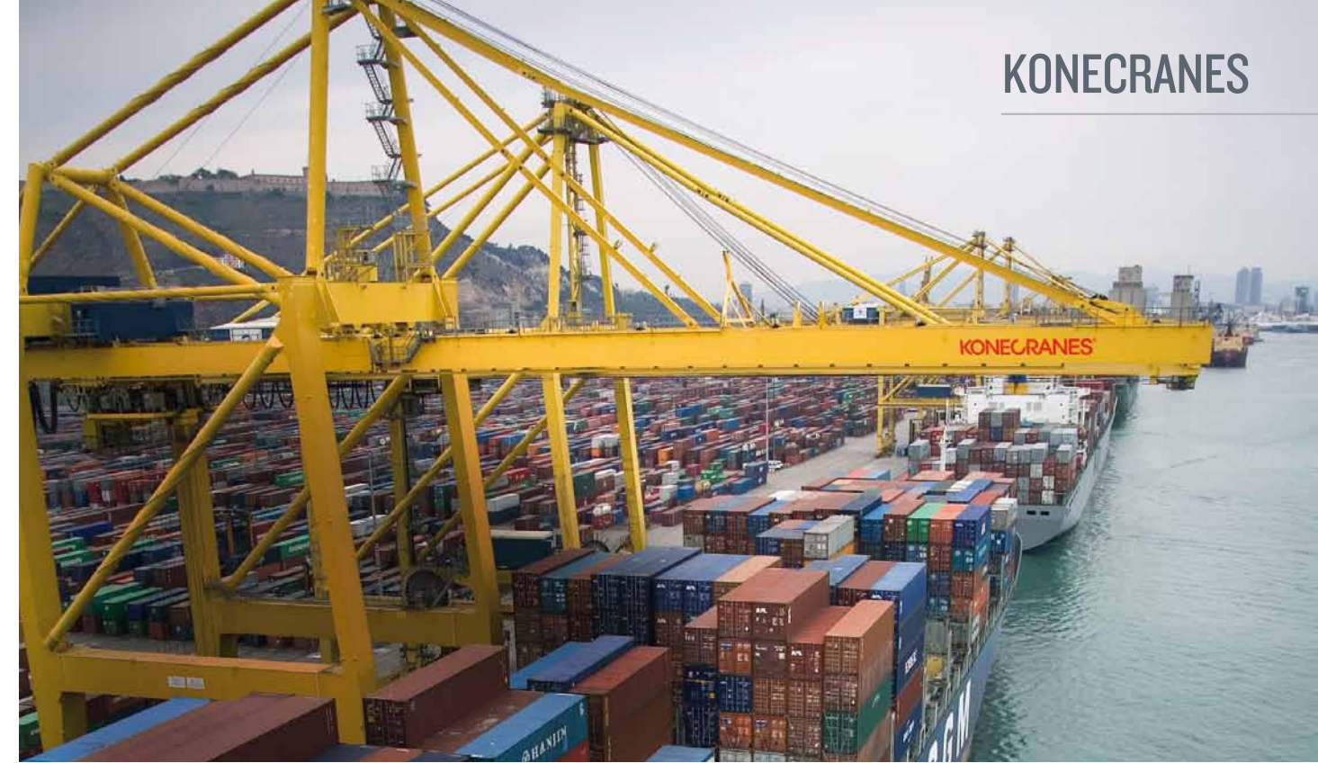
Ship-to-shore crane at Terminal De Contenidors Barcelona, Spain
