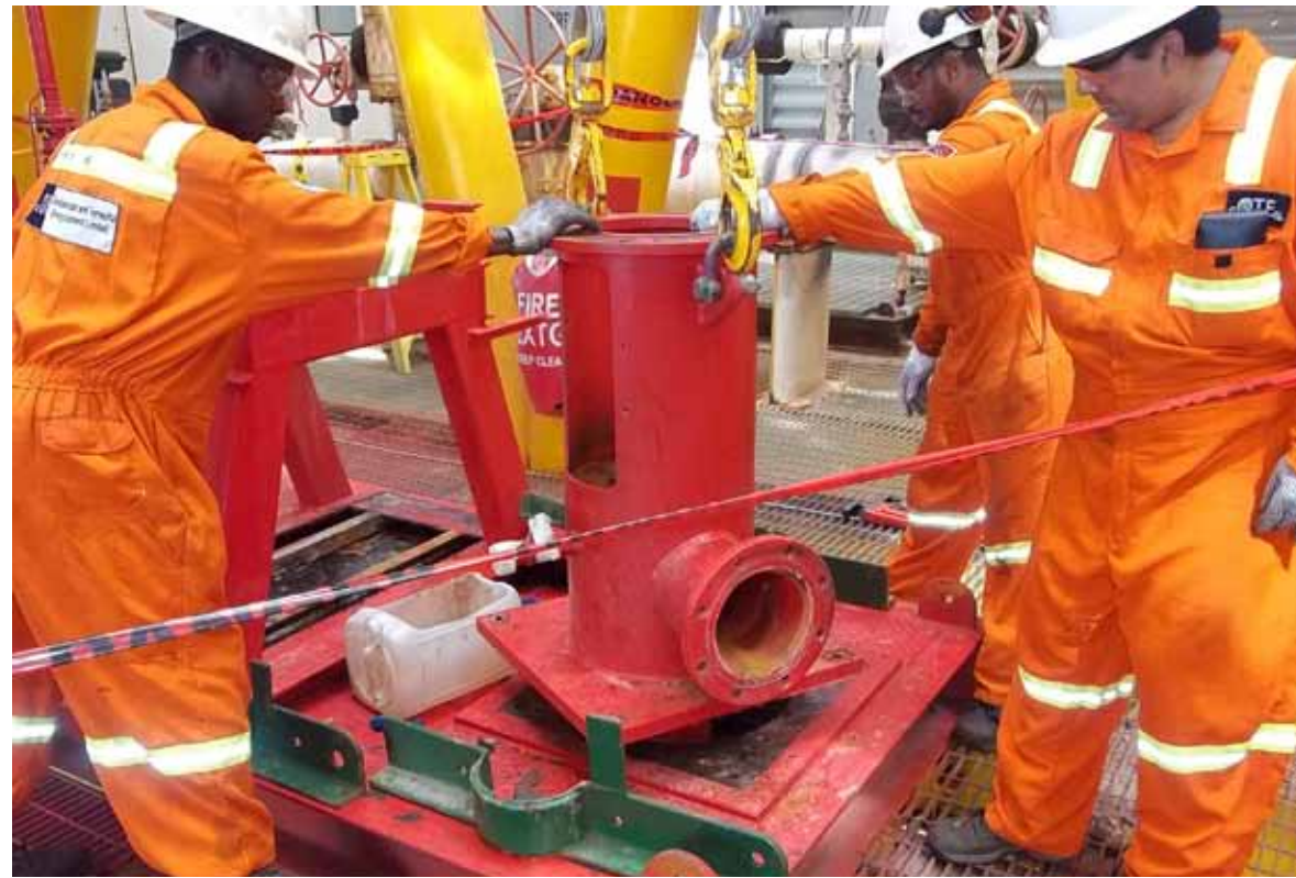
Overhauling and reinstalling a fire water pump on an offshore platform
