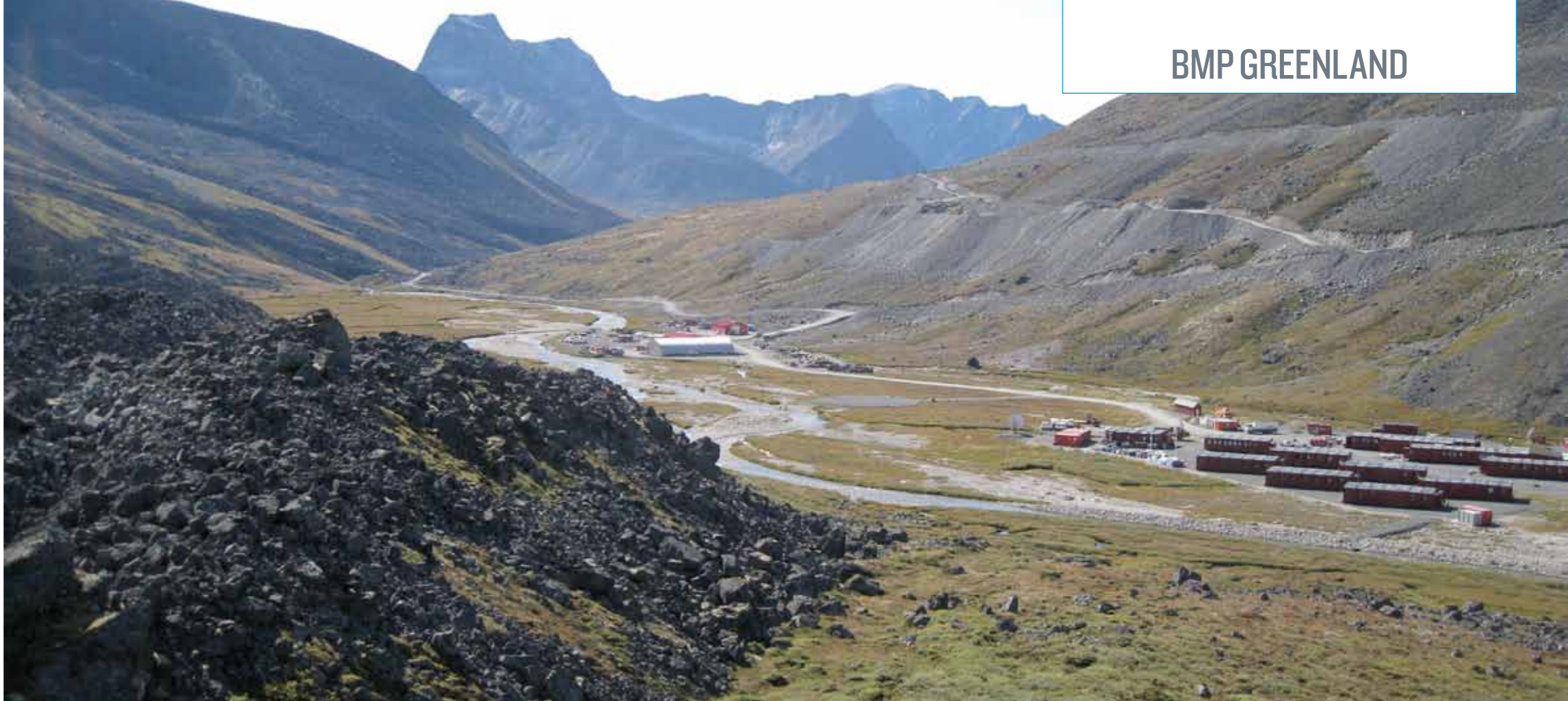
Nalunaq goldmine camp in South Greenland
