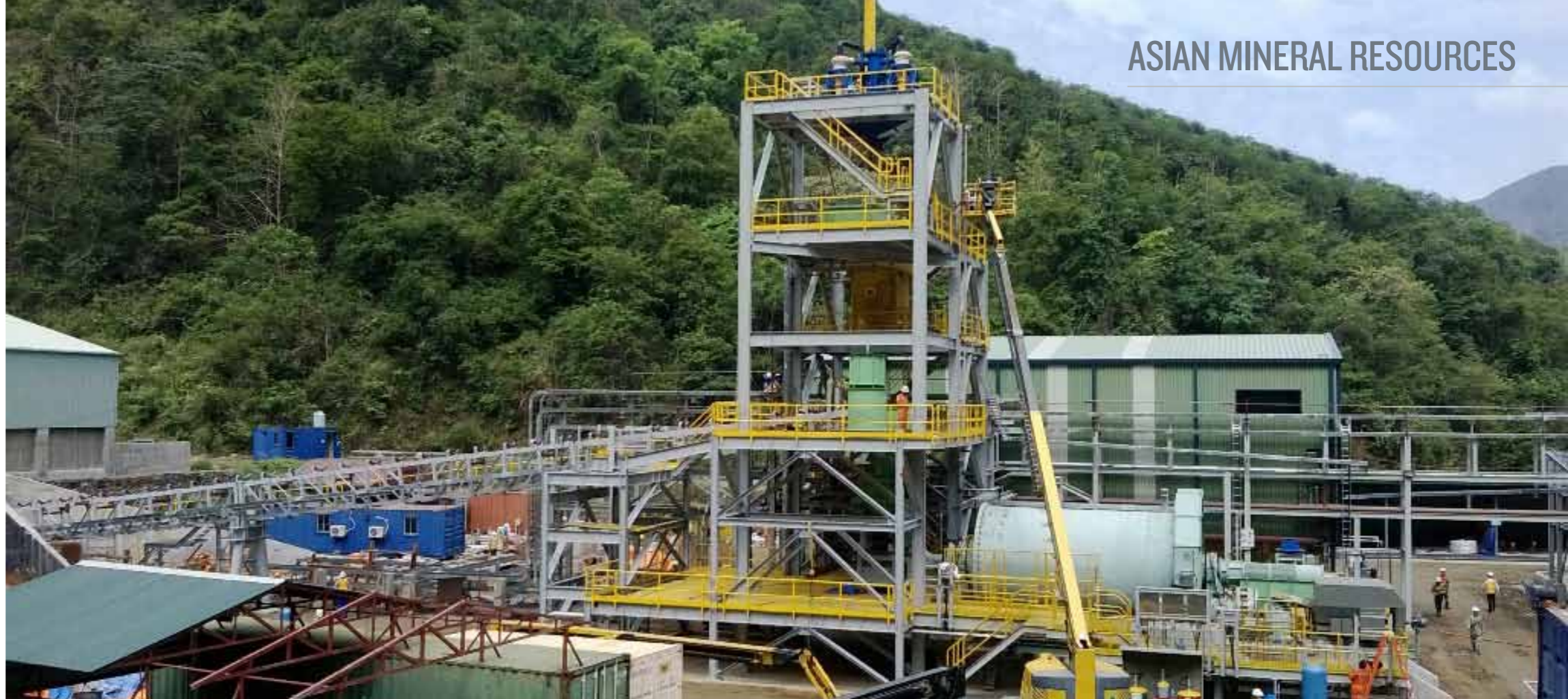
Overview of the plant site
