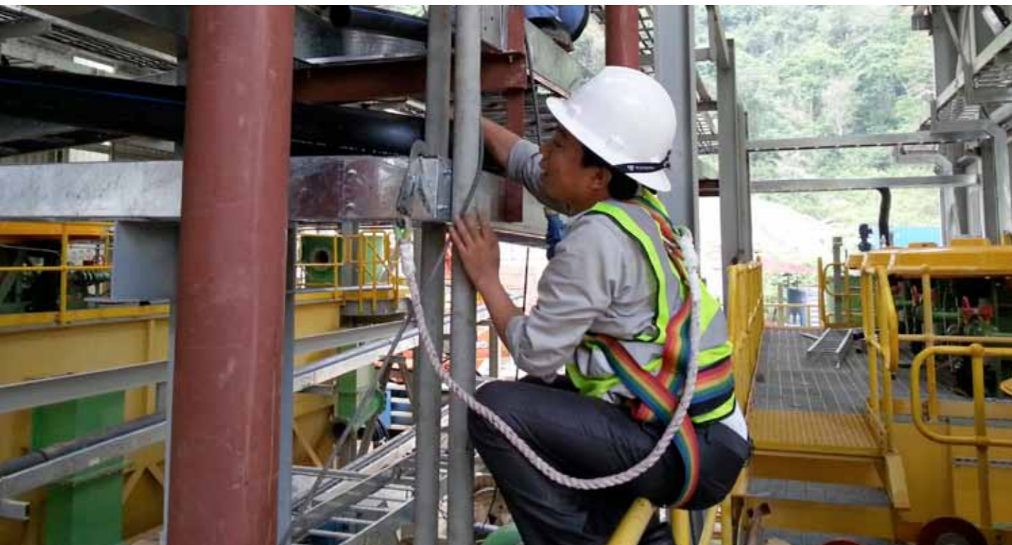
Plant worker carrying out maintenance
