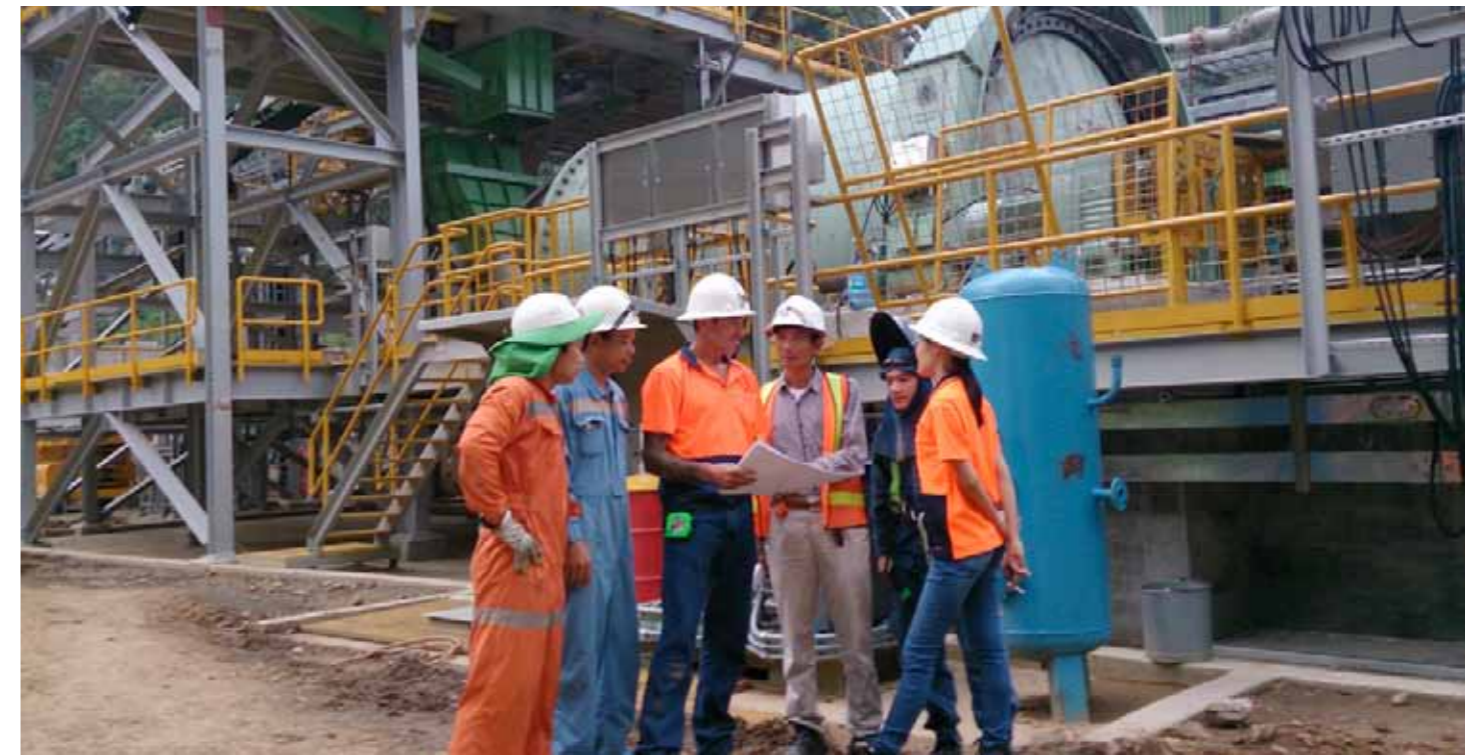
The next phase of construction being discussed
