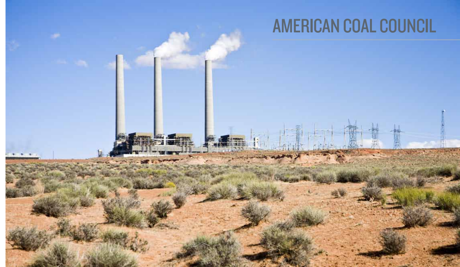
Coal-fired steam plant near Page, Arizona
