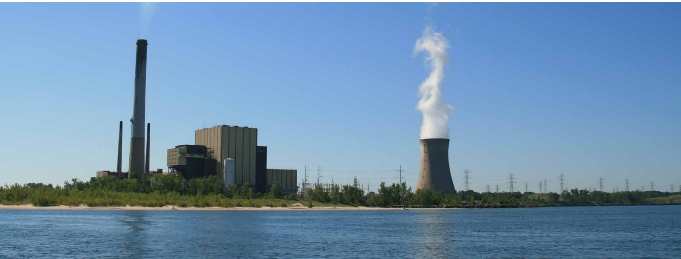
Power plant on Lake Michigan
